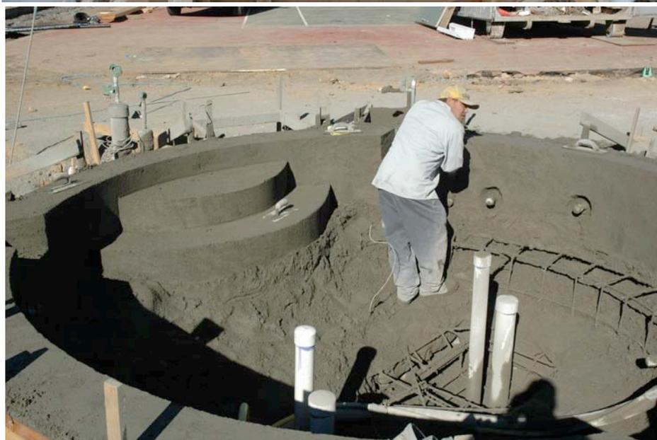
Gunite shot to form walls, floor and steps. Working leveling walls and cutting and shaping steps
