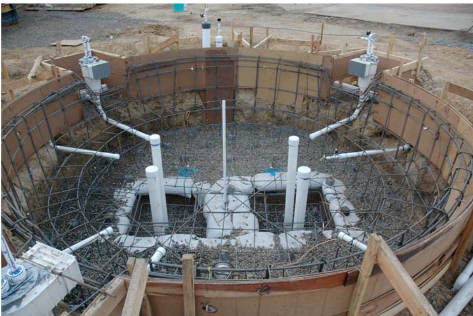
Skimmers, drains and inlets set, then the rebar is formed around the outside edge and bottom for strength
