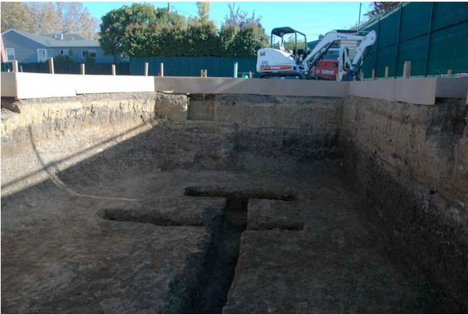
Shell of pool dug out, channels for pool lines in bottom
