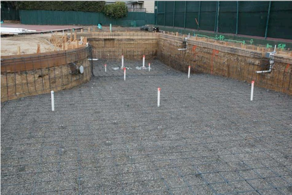
Rebar laid, water inlets sticking up through the bottom
