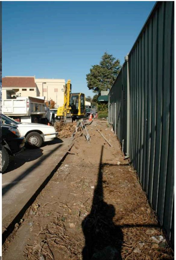
New sewer, water and storm drains line run outside of the building
